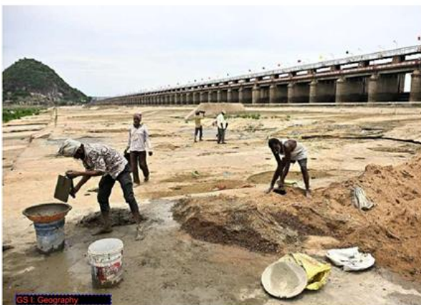
Labourers mix concrete and sand on the exposed Krishna riverbed in Vijayawada, for routine maintenance work during the seasonal low-flow period. The Prakasam Barrage is in the background. K.V.S. 088
